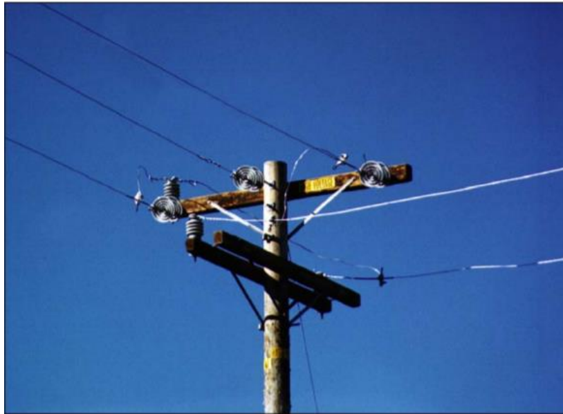
Figure 19: Illustrative example of a buck-arm junction pole
