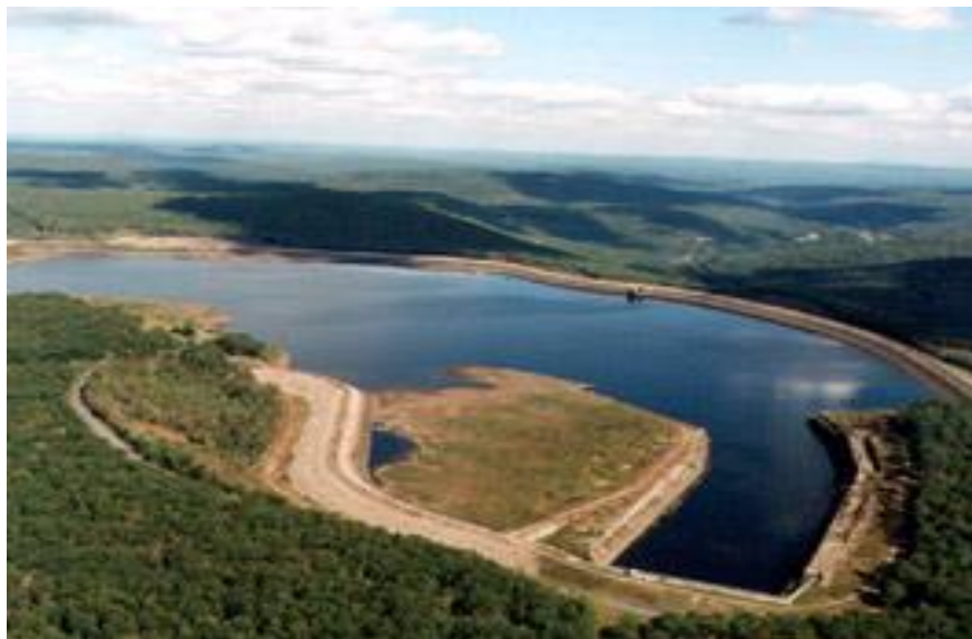
Figure 1-2: Northfield Mountain Pumped Storage Project in Massachusetts
