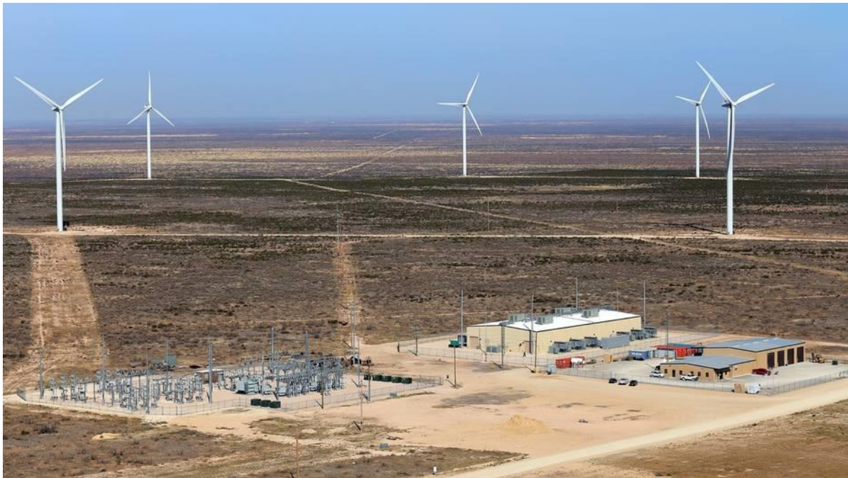
Figure 1-13: Duke Notrees Storage Facility in Texas
