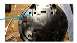
Inside of your meter box are two semicircular rings that now connect to nothing in the meter, therefore surge suppression no longer exists
