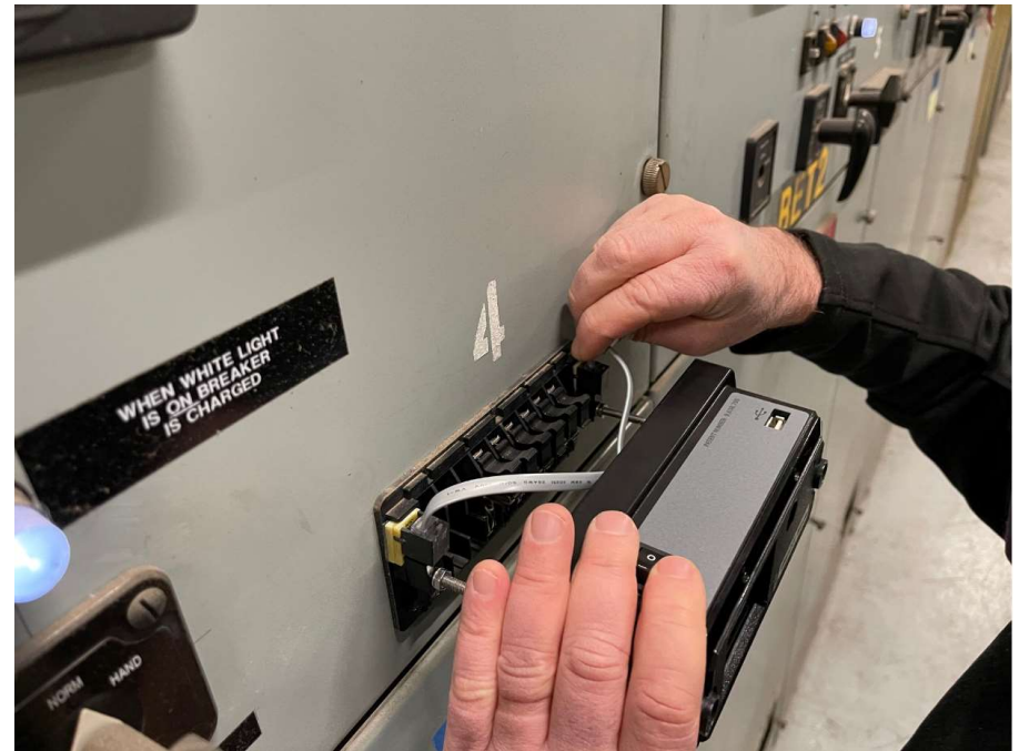
SMART Block Installation
