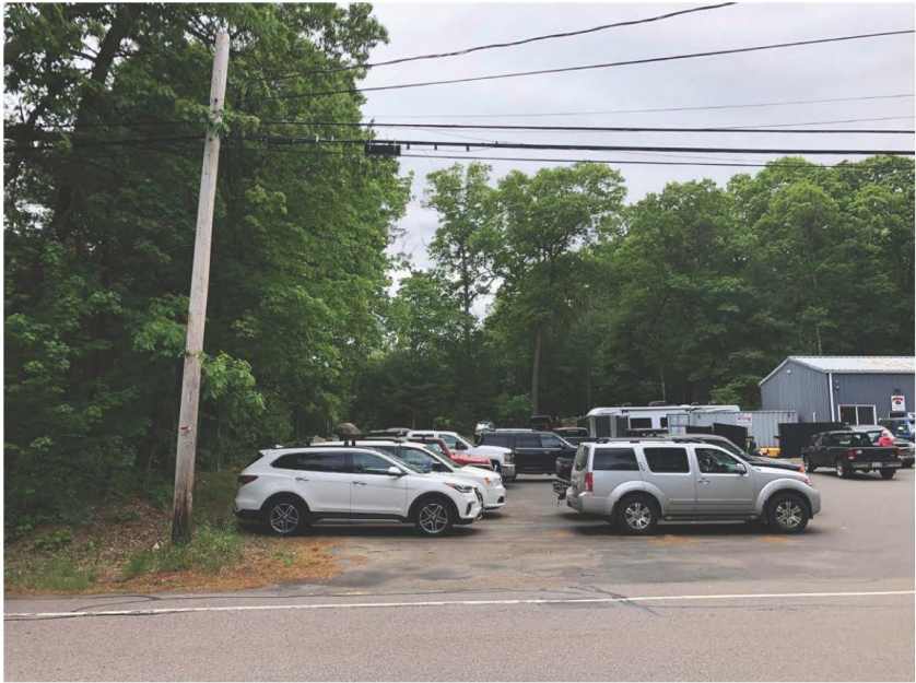
EXISTING VIEW Captured 5/28/2021
