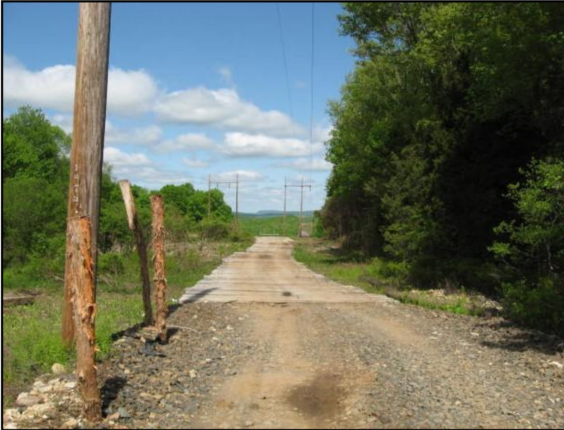
Construction mat access road.
