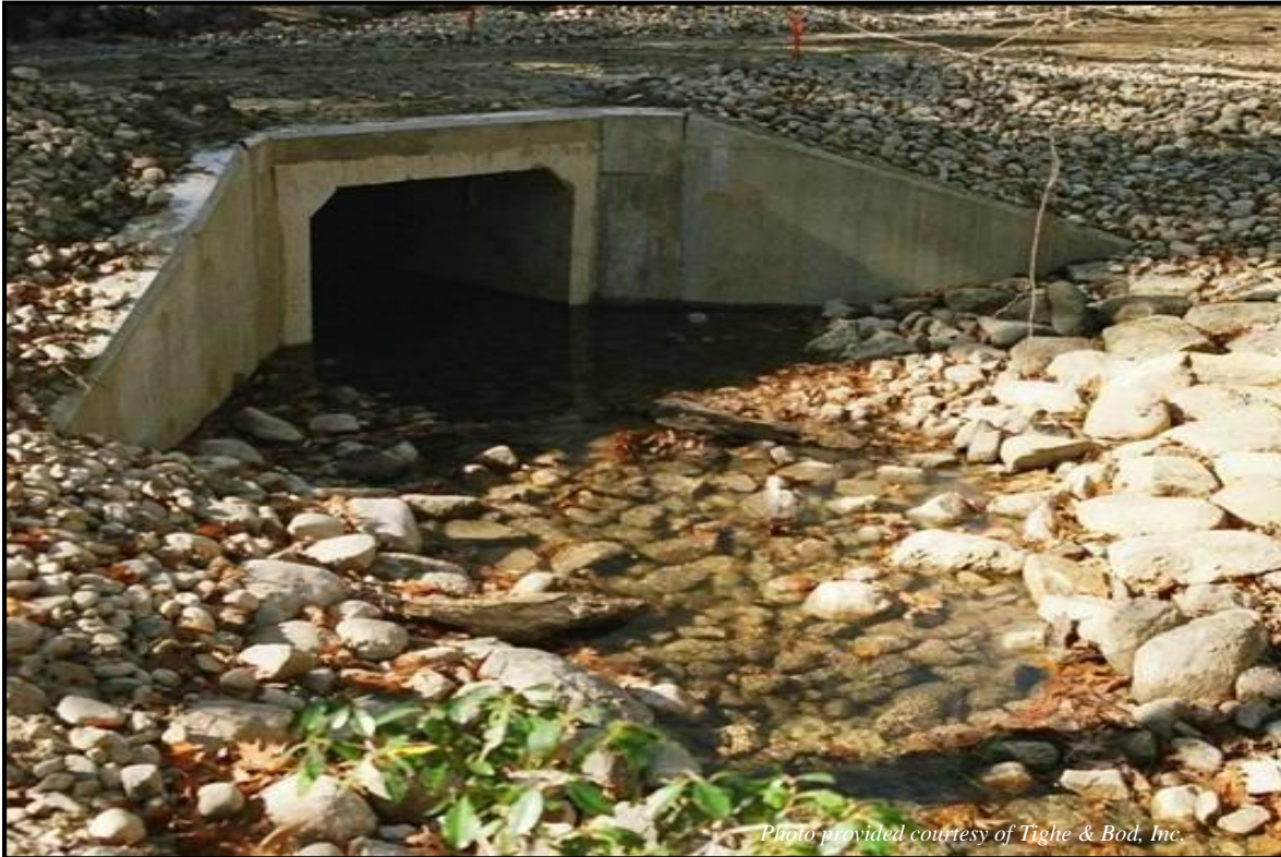
Embedded box culvert with wing walls.
