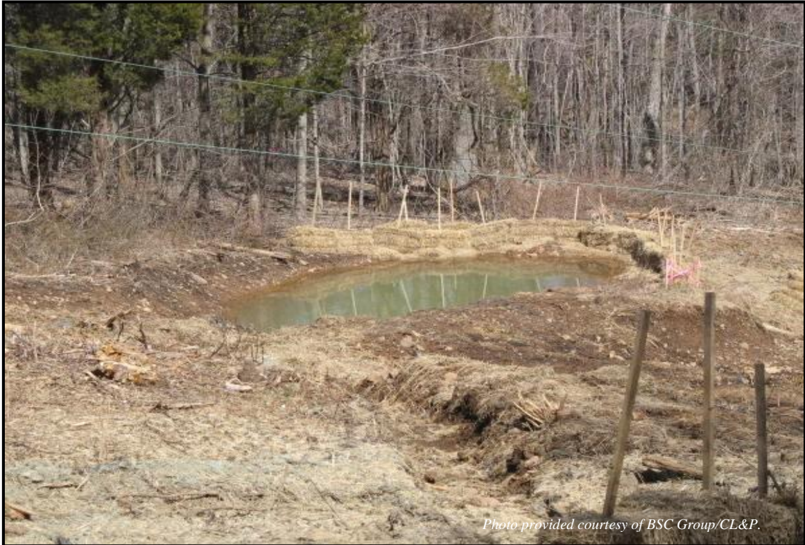
Sedimentation basin with hay bale filters.
