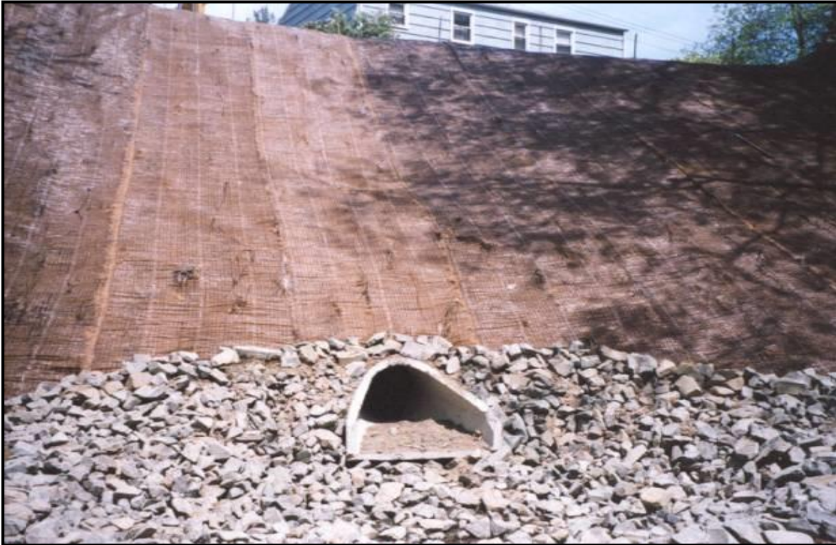
Pipe arch culvert.
