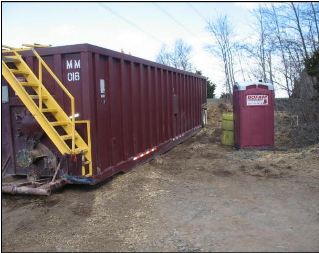
Frac tank on-site for dewatering activities.
