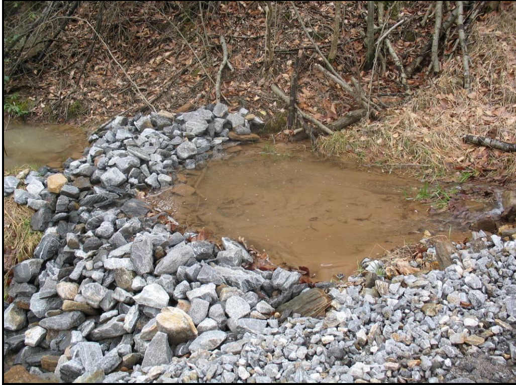
Stone check dam at construction site.
