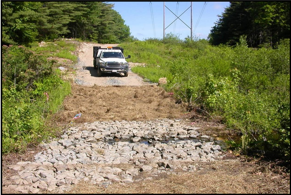
Intermittent stream crossing with angular stone.
