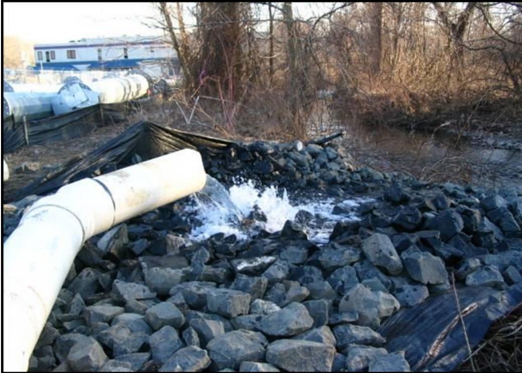
Riprap underlain by geotextile fabric
