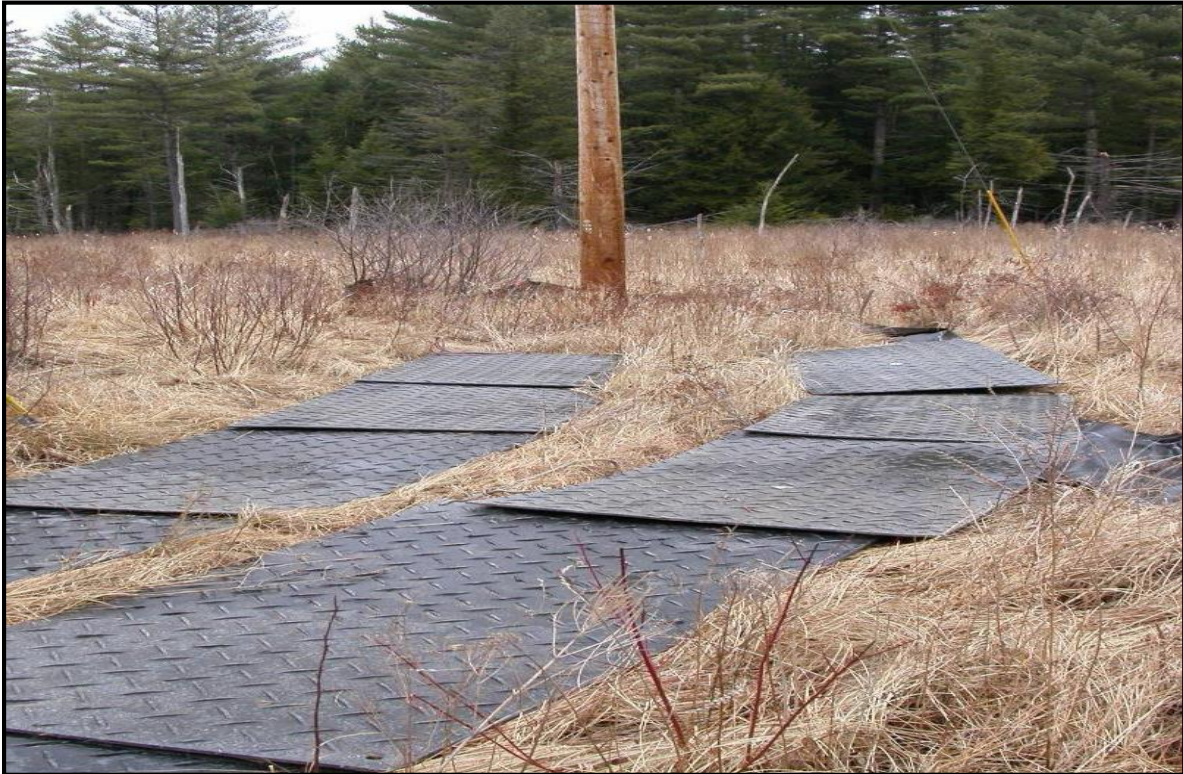
AlturMAT® tracks to utility pole in wetland.
