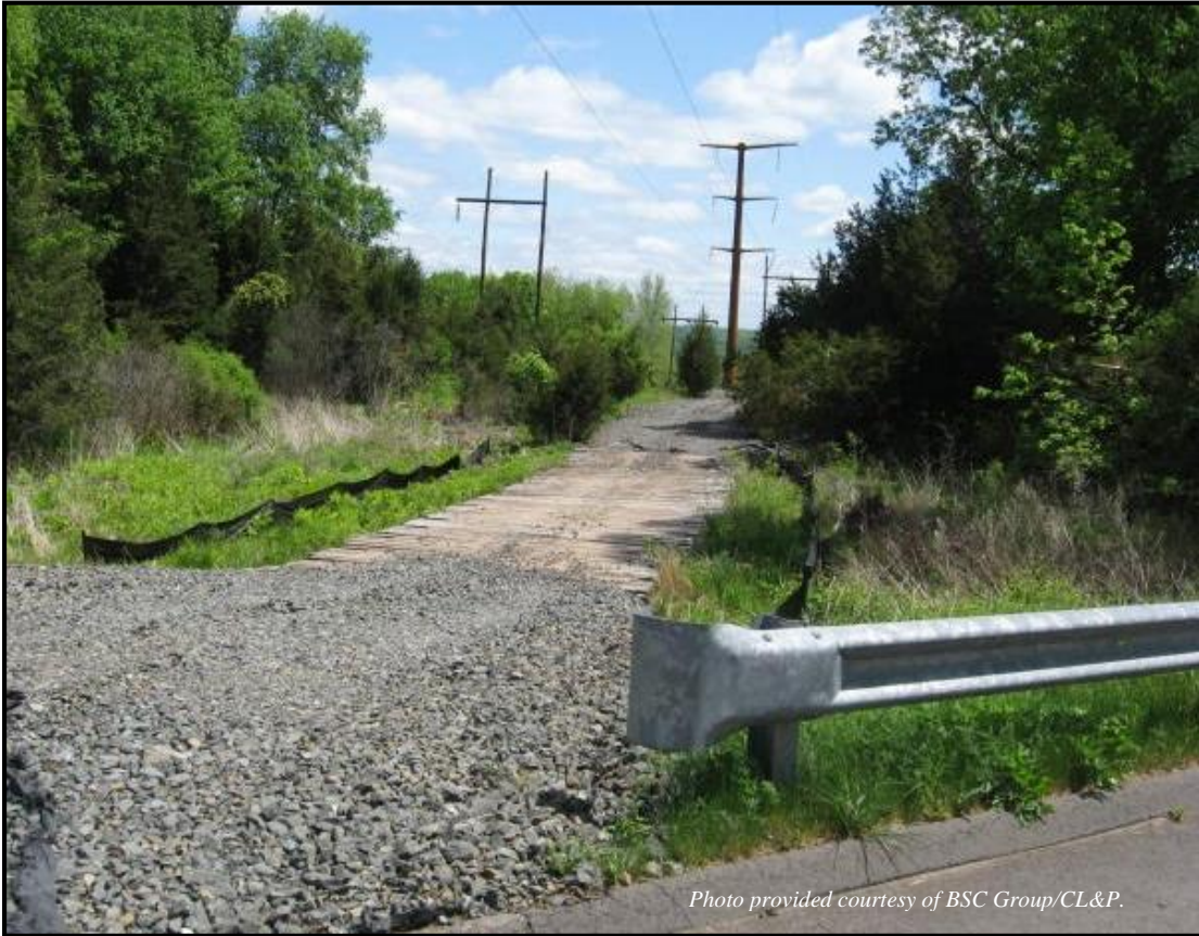
Construction entrance track pad.
