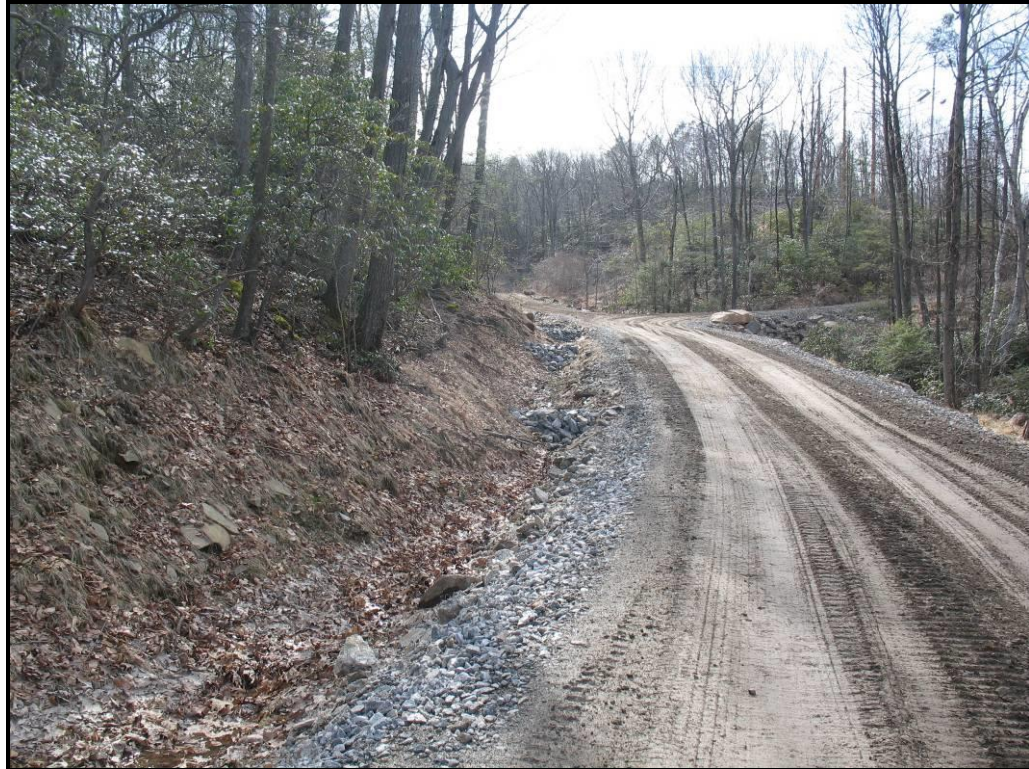
Stone check dams at construction site.
