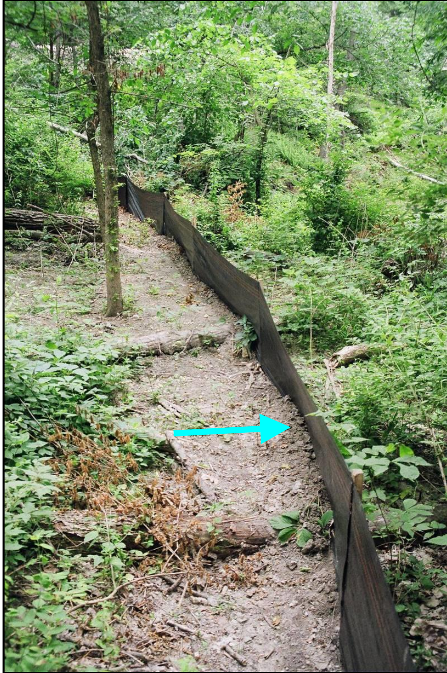
Properly installed and functioning silt fence. Direction of flow indicated by blue arrow.
