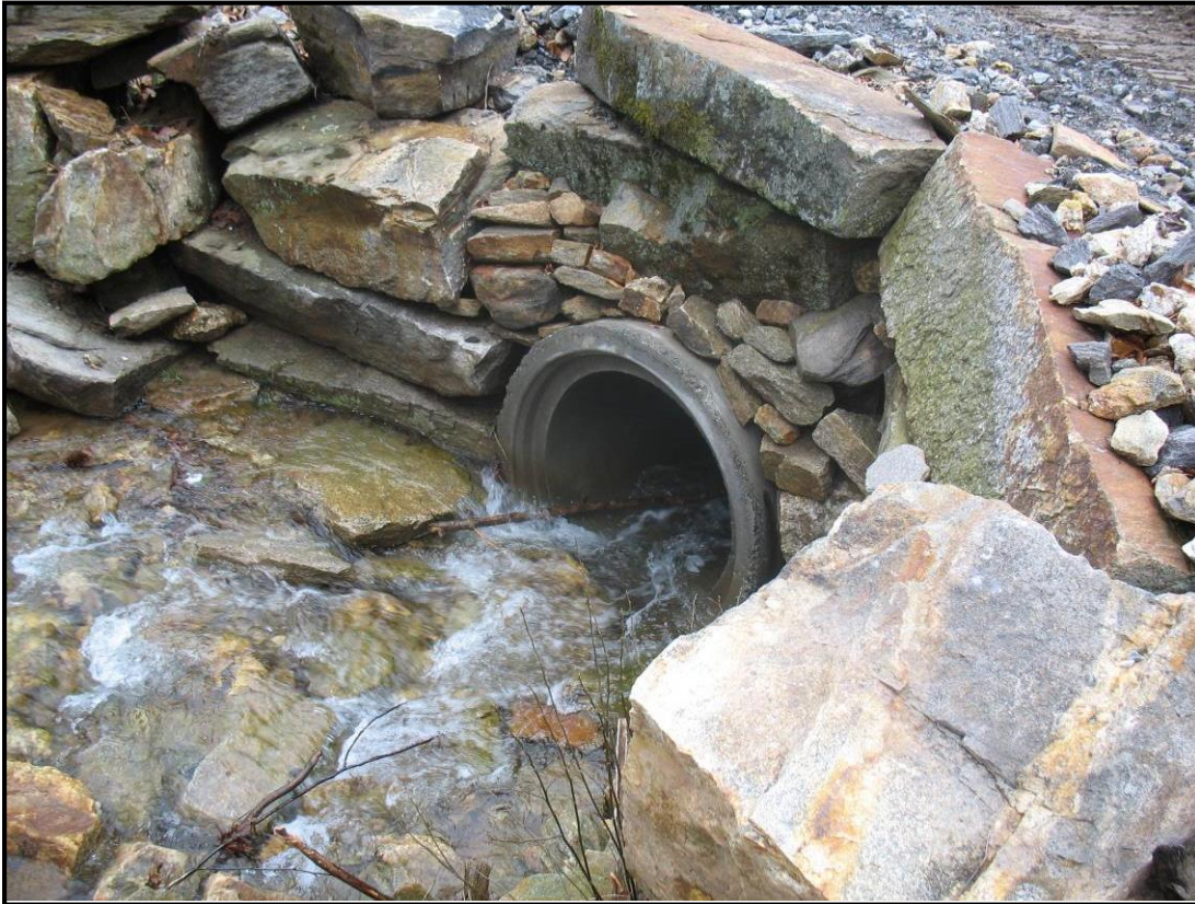
Culvert and riprap for stream crossing.
