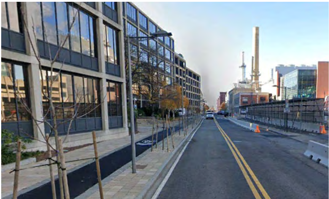
Photo 30: View facing south along Vassar Street. This portion is common to P11 and B29F West.
