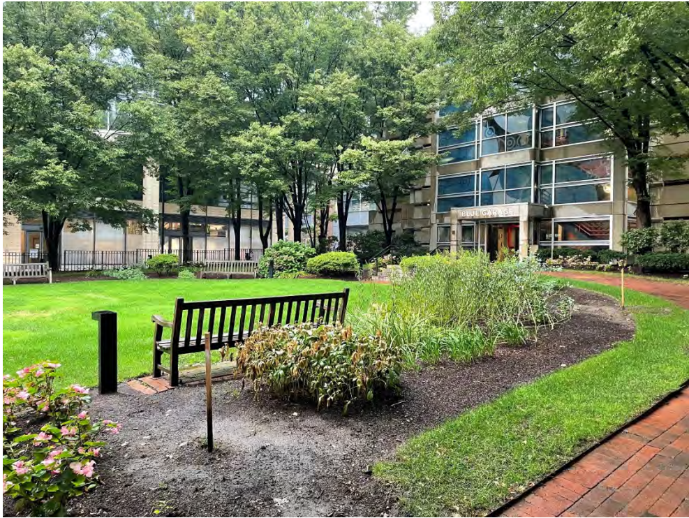
Photo 1: View facing northwest facing the proposed substation at the Blue Garage. This portion is common to all routes.
