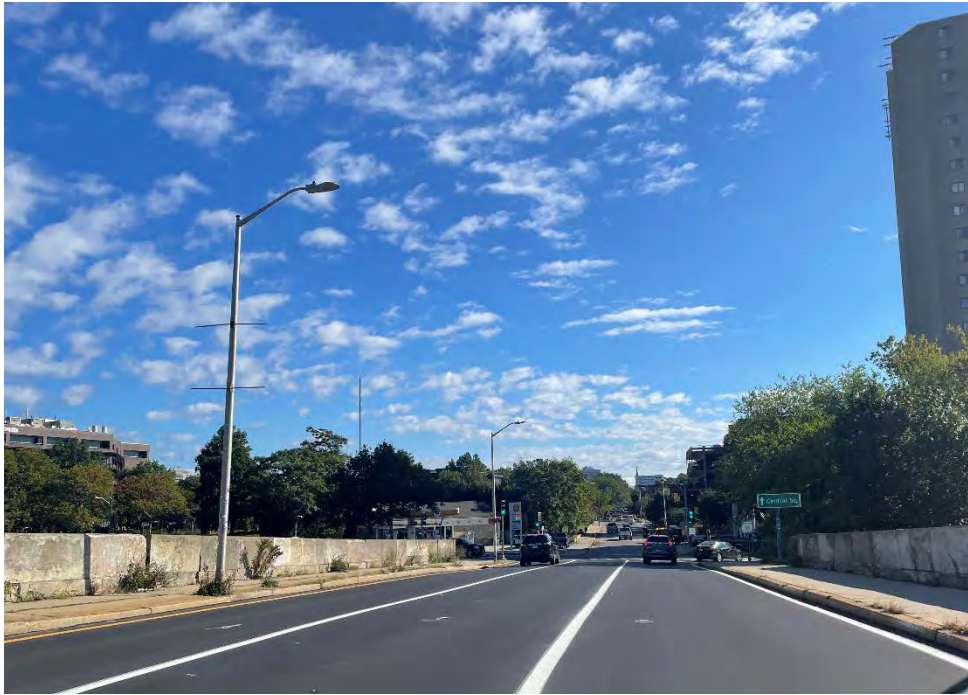
Photo 28: View facing northeast along the River Street bridge.
