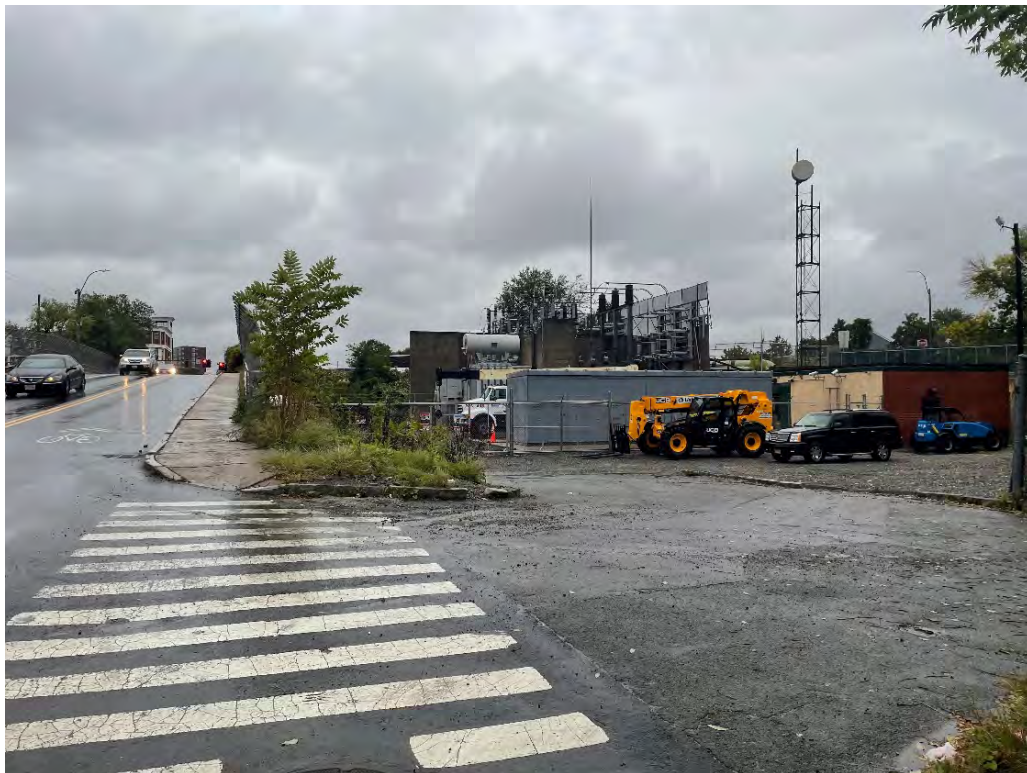
Photo 14: View facing south along Prospect Street looking into the Prospect Street Substation.
