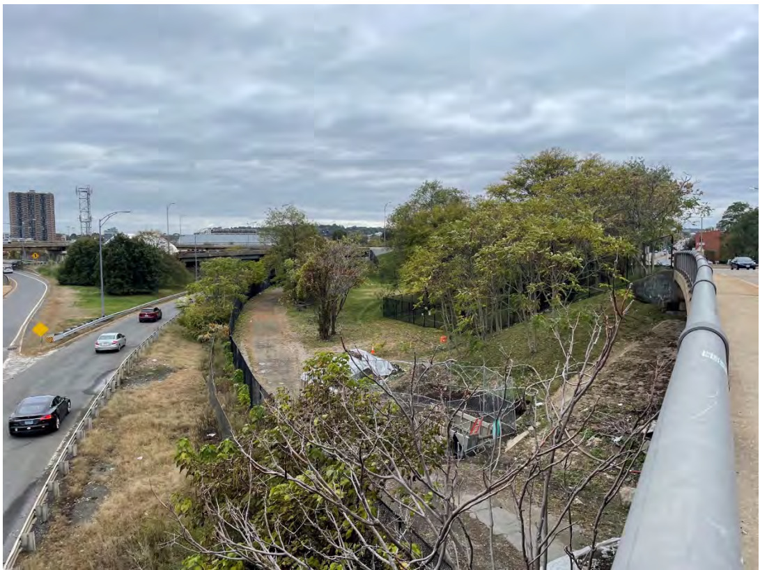
Photo 29: View facing east along Cambridge Street near the I-90 ramps. This area is common to B29F West and B31 East.
