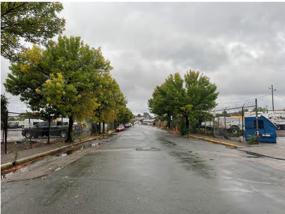
Photo 38: View of Linwood Street facing northwest.
