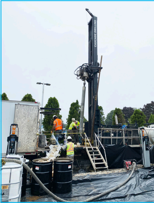
Figure 7. Pre-design drilling to gather more information about bedrock fractures
