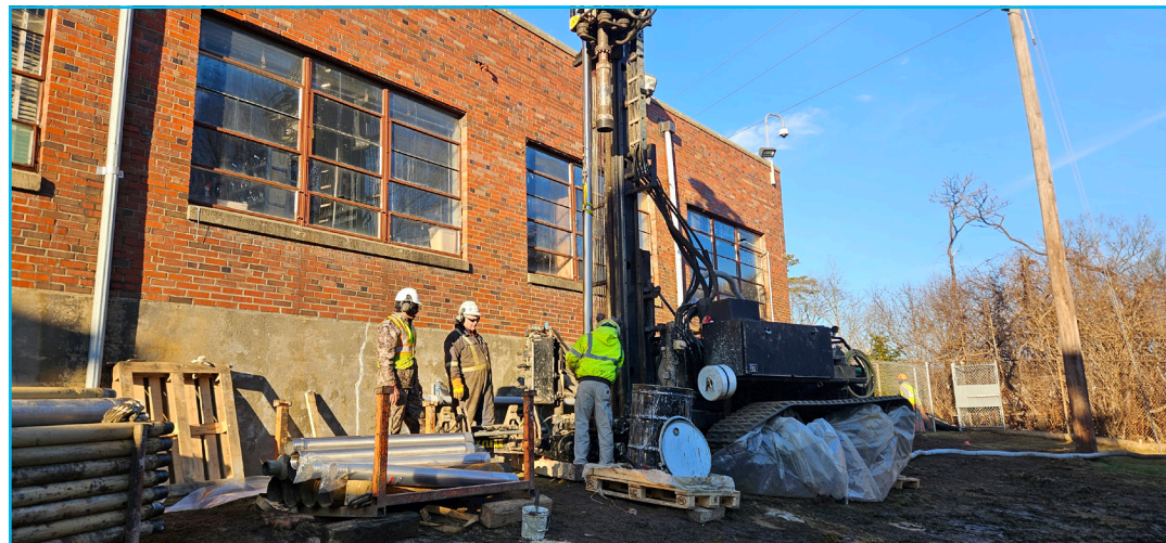
Figure 3. Drilling and installation of exterior thermal wells
