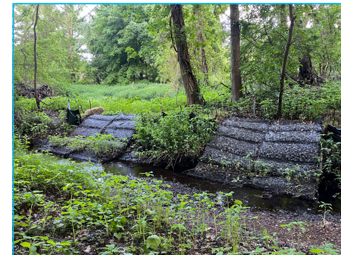
Figure 5. Stone covers reactive core mats along the stream
